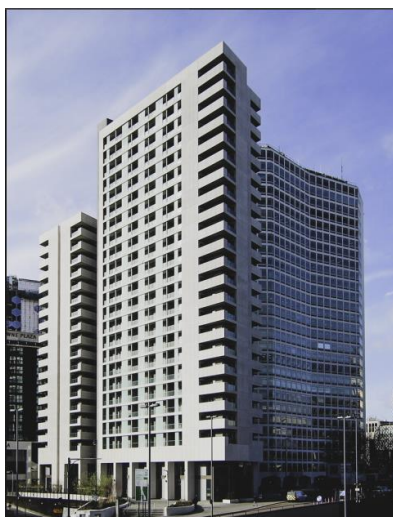
Figure 5 Precast concrete constructions, Arena Central, Birmingham, 2019 [13]
