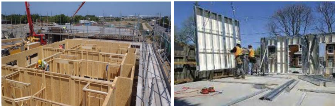
Figure 3 Timber walls [7]. Figure 4 Prefabricated Light Steel Framing [14]
